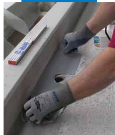
Laying flexible hyphalon brace
