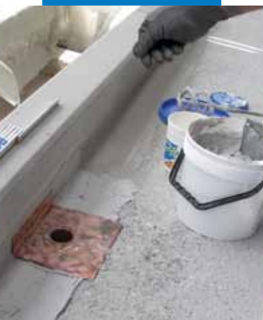
Laying a copper neck-flange and drain spout
