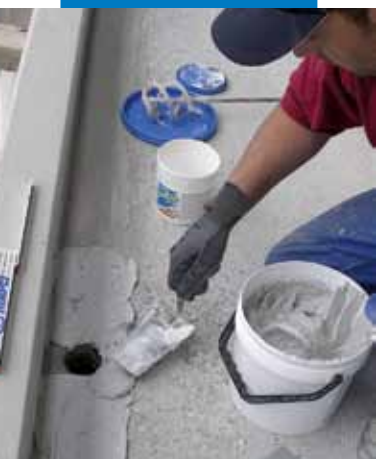
Applying Adesilex PG4 with a trowel
