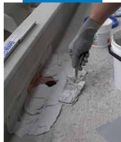
Subsequent smoothing with Adesilex PG4
